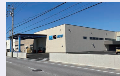
Exterior view of Hostec factory
